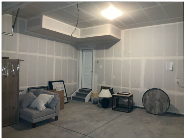
Personal items in garage block complete inspection of all floor, wall and ceiling areas.
