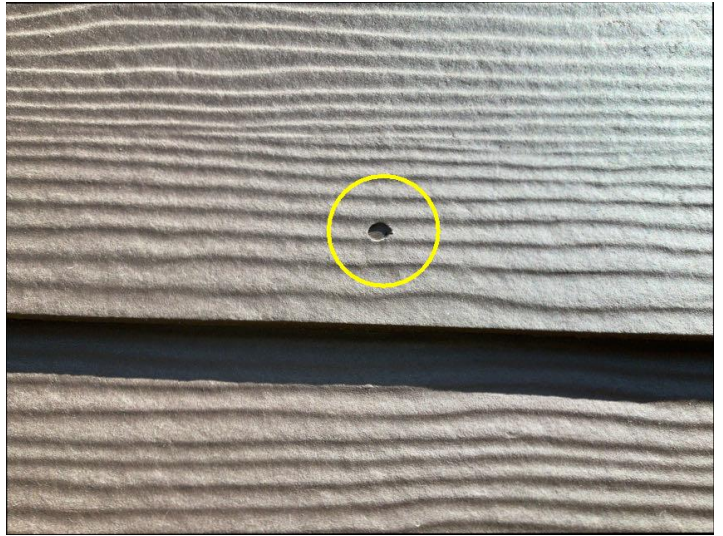
Some siding nails are protruding through the siding. This condition can allow moisture intrusion, damage to the siding material, and reduce the overall effectiveness of the exterior cladding. Recommend repair or adjustment by qualified contractor to help maintain siding, integrity and weather resistance.
