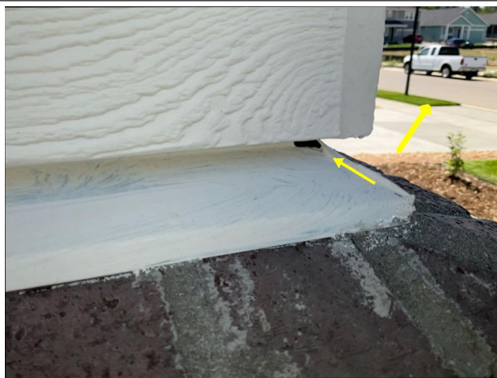
Caulk and seal all gaps, cracks and openings.
