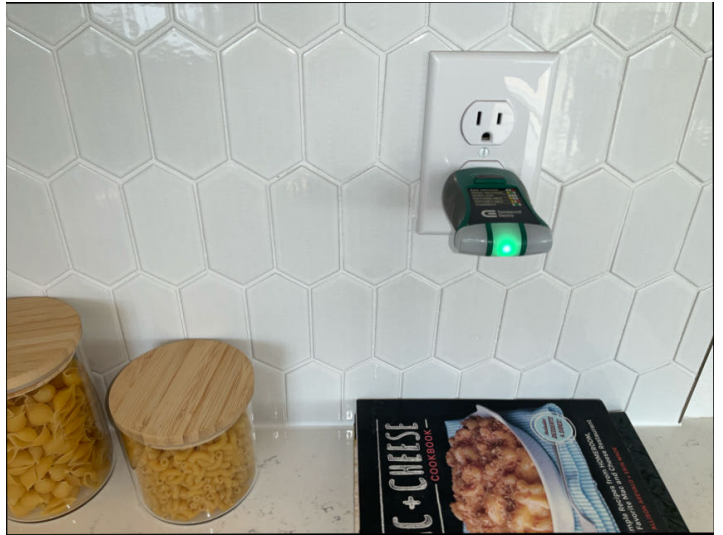
Kitchen GFCI reset is in electrical panel box.
