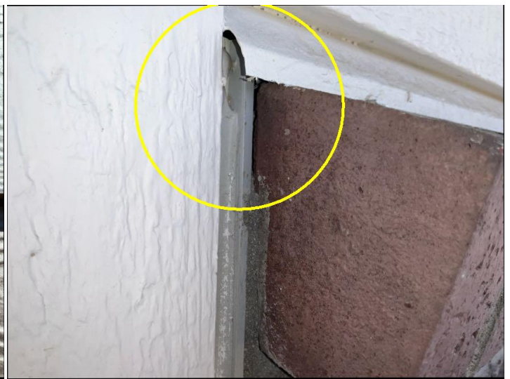
Caulk and seal all gaps, cracks and openings.
