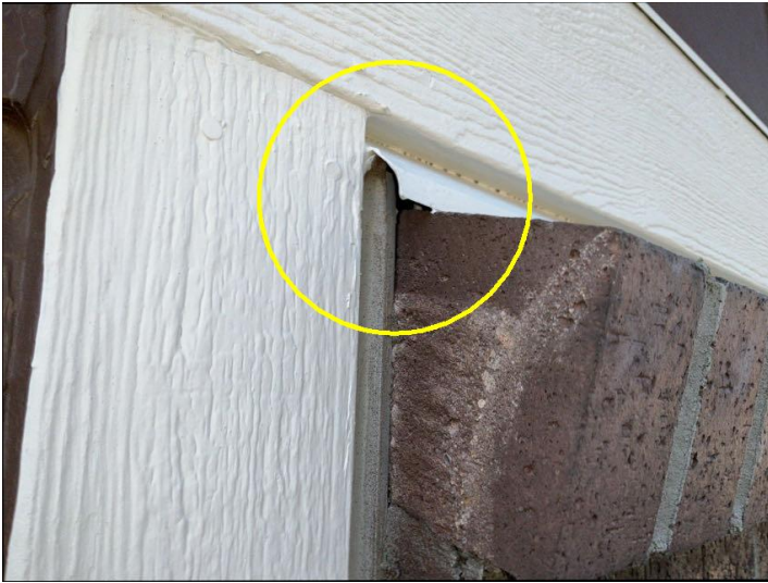
Caulk and seal all gaps, cracks and openings. Left side of house just past front porch.
